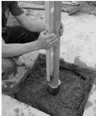
Checking post is vertical
