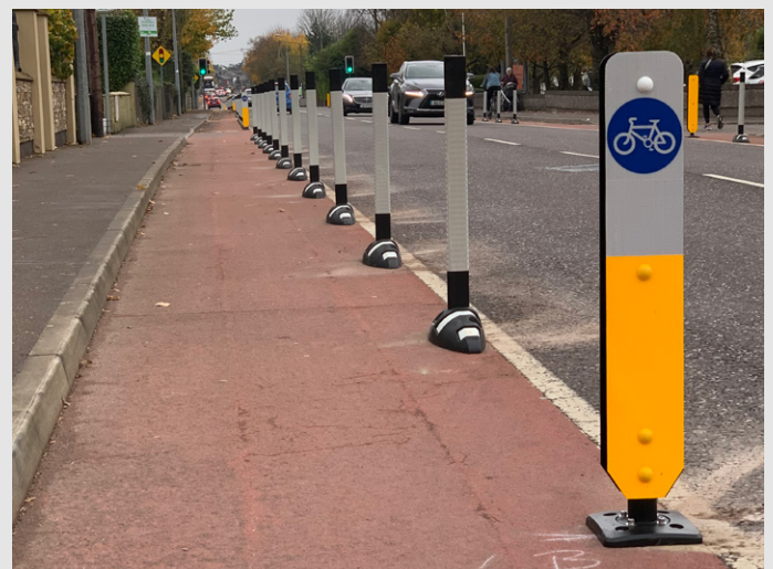
Tiger Wands used in conjunction with Hazard bollards for enhanced cycle lane delineation
